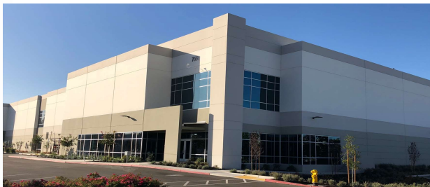
New Livermore Manufacturing Center
