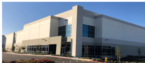
New Livermore Manufacturing Center
