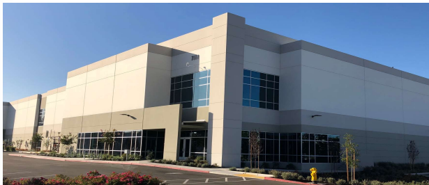
New Livermore Manufacturing Center
